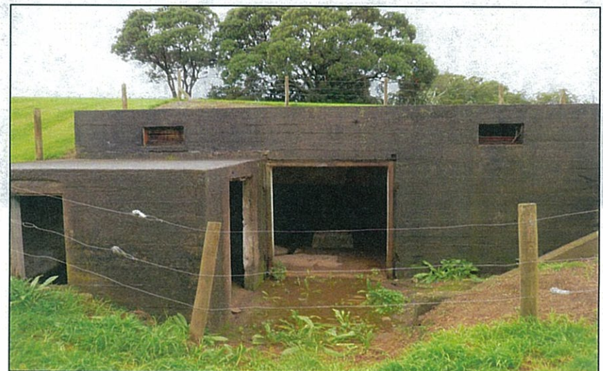
PHOTO 13 (Bottom): The electrical generator bunker (2010)
