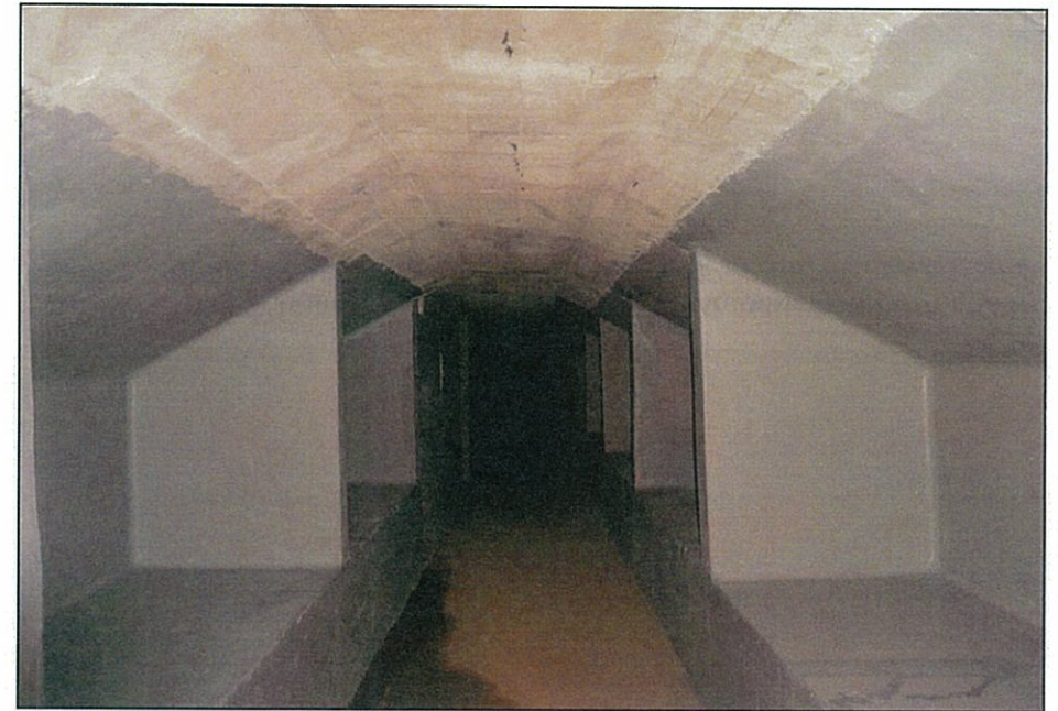
PHOTO 12 (Top): Shell storage niches in the passage connecting the gun emplacements (2010)
