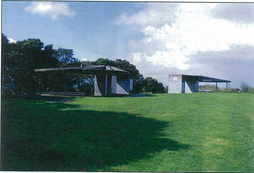
PHOTO 10 (Top): The Red Bluff gun emplacements stripped of their camouflage facades (2010)
